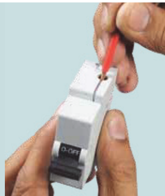
Connect the outgoing phase wire on upper terminal & tight it
