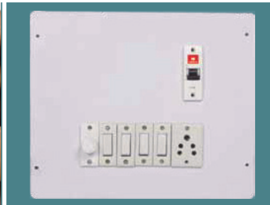
Mini MCB is successfully installed
